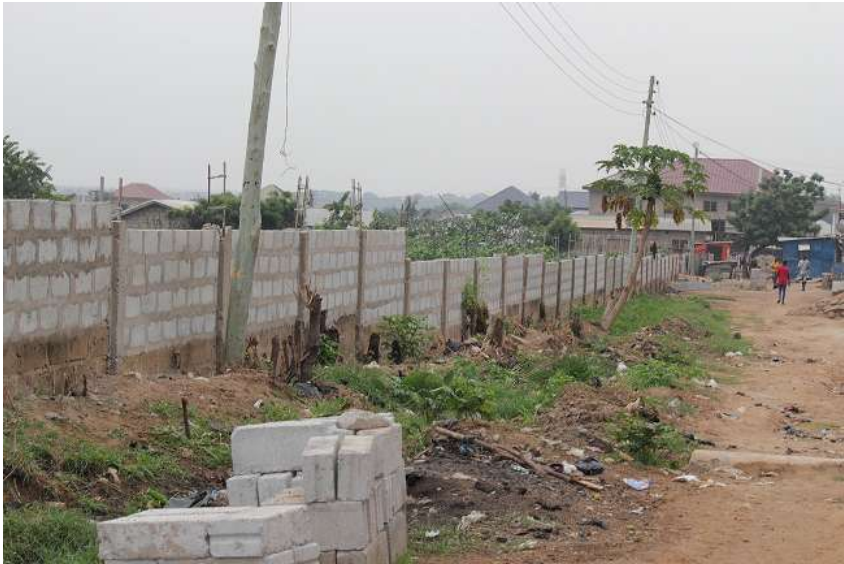
Back-wall Hopeland compound.
