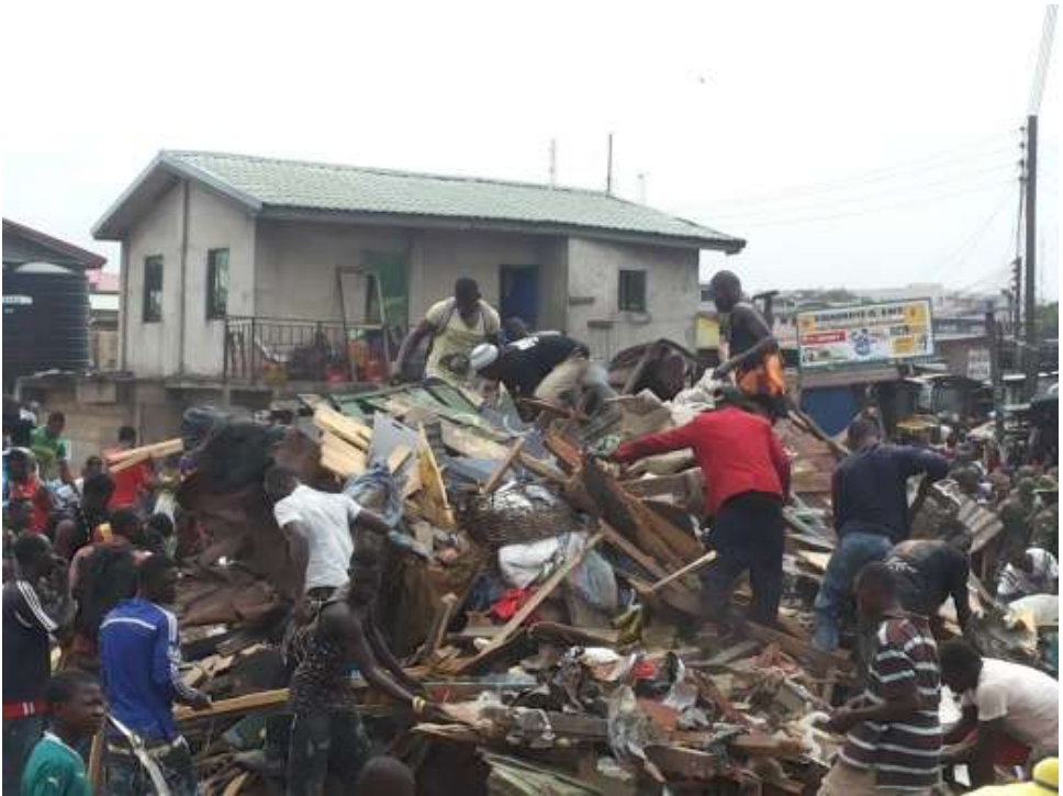
Demolishing of part of Old Fadama.
