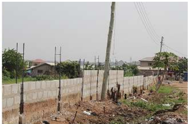
New fence wall
