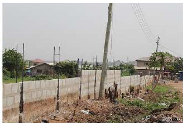
New fence wall
